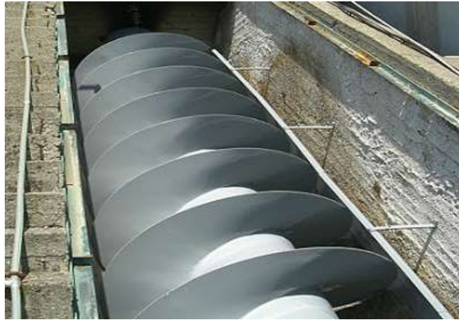
Figure 23 – CLOSE UP VIEW OF AN ARCHIMEDES SCREW PUMP.
