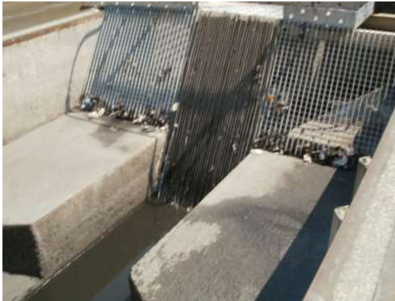
Figure 2 – A TYPICAL HAND-RAKED BAR SCREEN.
