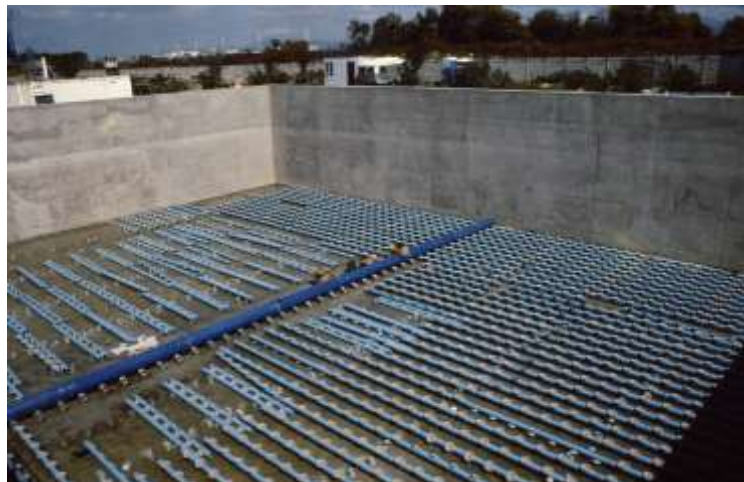
Figure 31 – FINE BUBBLE DIFFUSER FLOOR LAYOUT (Under construction)
