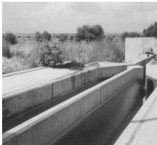
Figure 6 – A TYPICAL HORIZONTAL GRIT CHANNEL PAYOUT.
