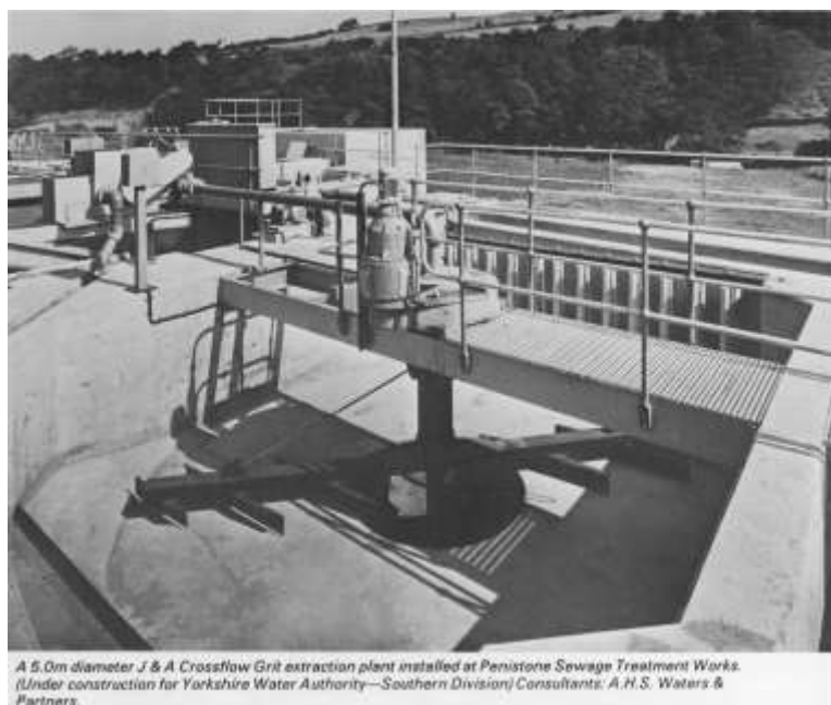
Figure 9 – HORIZONTAL FLOW GRIT TANK.
