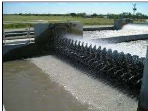
Figure 33 – EXAMPLE OF HORIZONTAL SHAFT SURFACE AERATOR.
